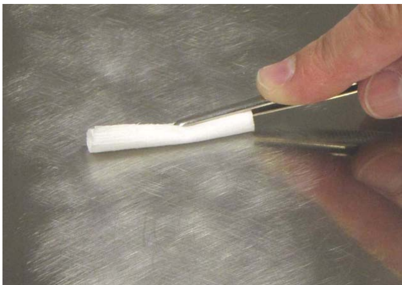
Fig. 2.4: Cleaning the roughened installation surface
